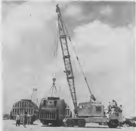
A CONDENSER is a big load for any crane. Help from the crane was needed to unload the machinery at the Balashi work scene; no group of men could wrestle the heavy and awkward machinery around.
